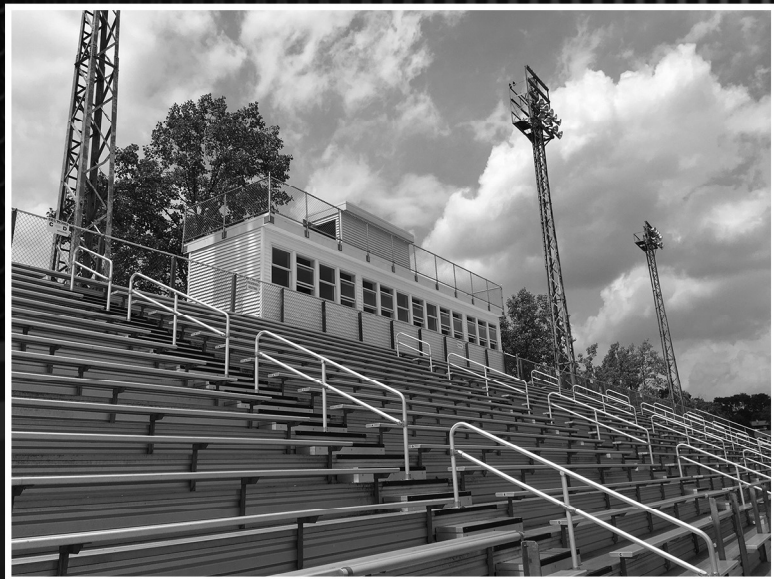
Selinsgrove Football Field Pressbox Design & Light Inspection
