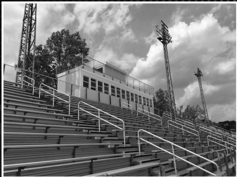
Selinsgrove Football Field Pressbox Design & Light Inspection
